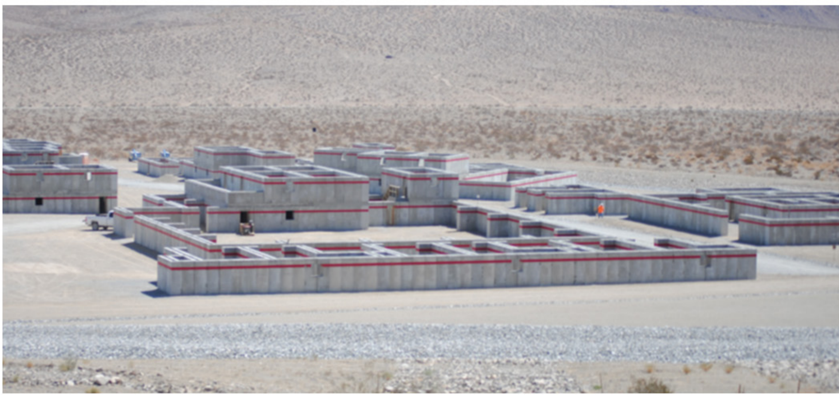
Live-Fire Training Village (10 buildings total , 2 two-story structures)
